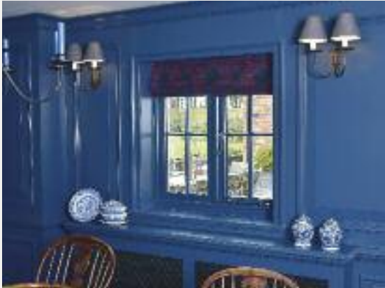
Cottage casement window finished in a colour complementary to Fired Earth 'Carbon Blue', featuring a Polished Nickel Reeded handle and matching pegstay.
