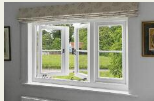
Flush casement windows finished in 'French Grey' externally and a colour complementary to Farrow & Ball 'Wimborne White' internally, with 18mm astragal glazing bars. Manufactured in Engineered Meranti Hardwood.
