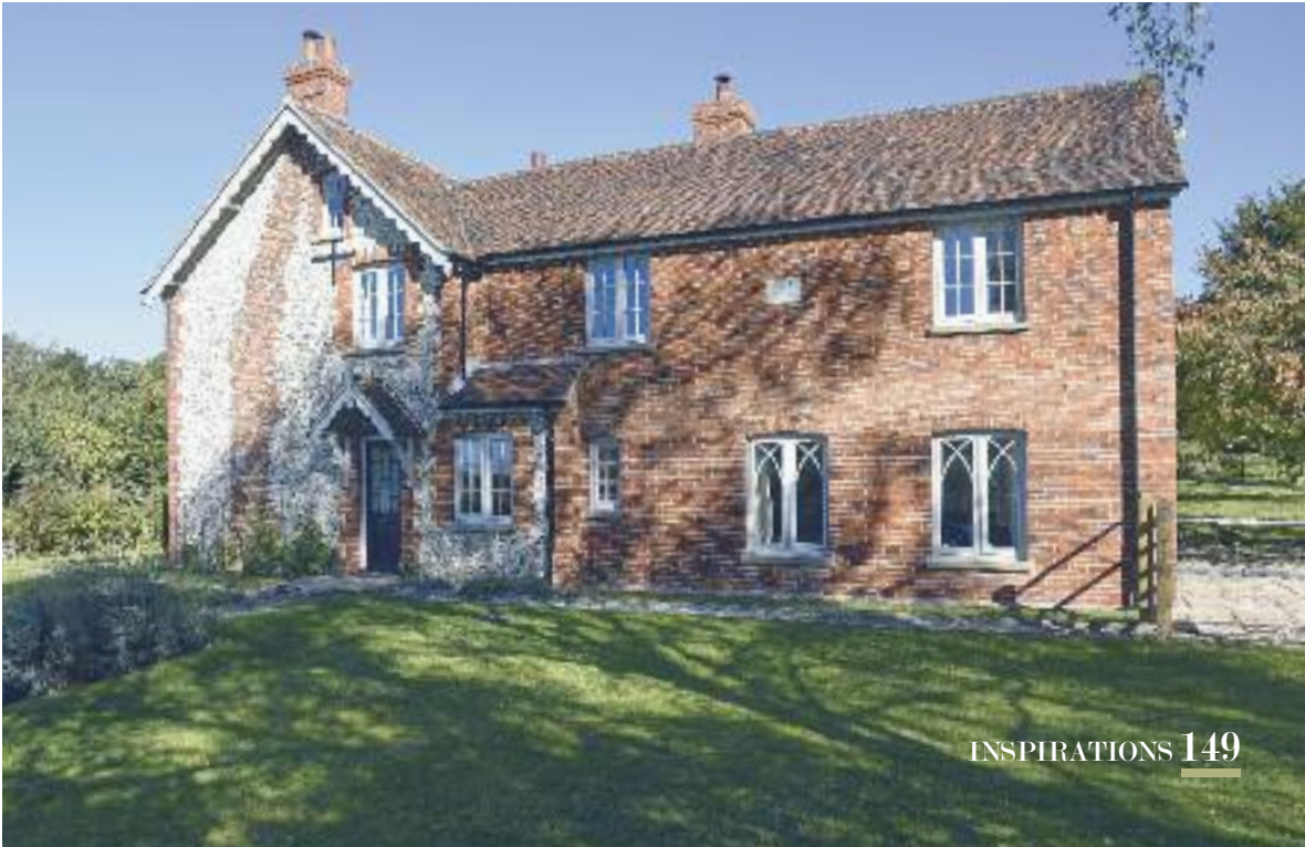
Flush casement windows finished in 'Porcelain' externally and 'White' internally with regular and gothic style 27mm astragal glazing bars and featuring Antique Brass Unlacquered Contour handles and pegstays from Samuel Heath.
