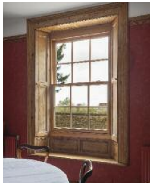
Slim sash windows with 18mm astragal glazing bars, and hung on traditional cords and weights. Finished in a colour complementary to Farrow & Ball “White Tie” externally with some in a “Light Oak” stain internally. Manufactured in Engineered European Redwood.
