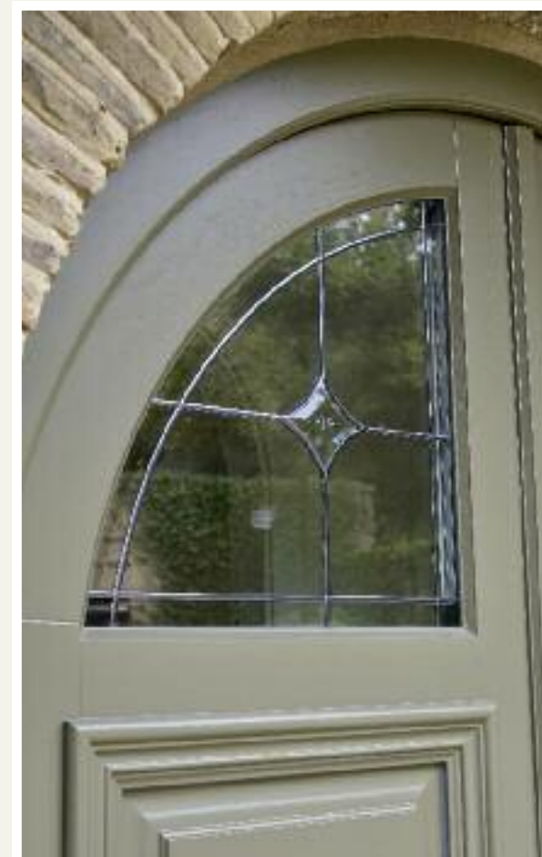
Bespoke, arched Hillingdon double entrance door finished in ‘Oxford Clay’ with Bevel leaded glazing design and an Antique Brass Unlacquered Profile Shoulder handle from Samuel Heath. Manufactured in Engineered Meranti Hardwood.
