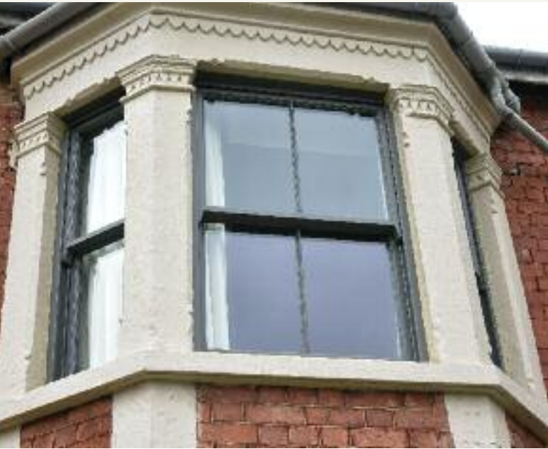
Slim sash windows finished in 'London Grey' with decorative sash horns including variations with vertical 18mm astragal glazing bar.
