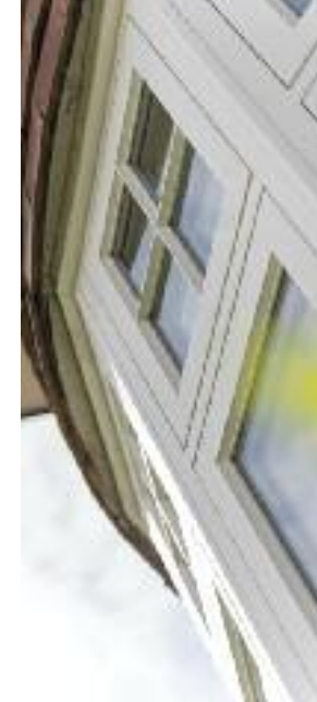
Flush casement windows finished in 'Off-White', with 18mm astragal glazing bars. Manufactured in Engineered European Redwood.
