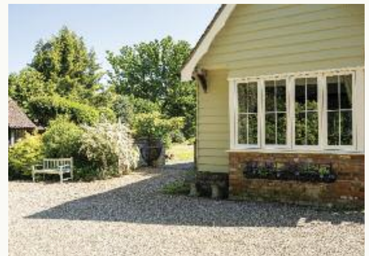
Flush casement windows in "Canvas" with 18mm astragal glazing bars. Manufactured in Engineered European Redwood.
