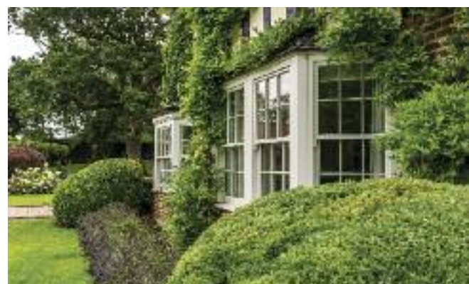
Slim sash windows, casements and arched French doors in a range of configurations, all in the colour “Smoke Cream” externally with 18mm astragal bars.
