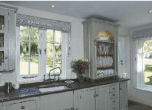
Flush casement windows finished in 'Porcelain' externally and 'White' internally with regular and gothic style 27mm astragal glazing bars and featuring Antique Brass Unlacquered Contour handles and pegstays from Samuel Heath.
