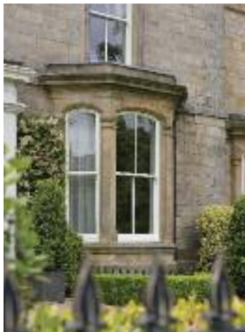
Slim sash windows with chains and weights mechanisms, featuring 18mm astragal glazing bars, all finished in a colour complementary to Farrow & Ball "All White". Manufactured in Engineered Meranti hardwood.
