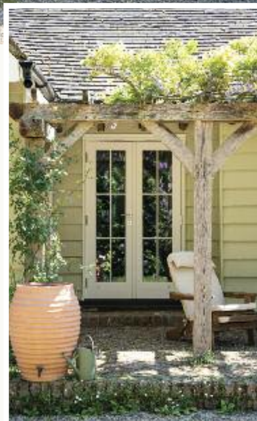
French doors finished in "Canvas" with 18mm astragal glazing bars. Manufactured in Engineered European Redwood.
